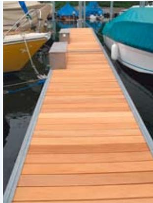
A refurbished system with new floats, these guarantee safe, long-term buoyancy. The new surface completes the picture. An economical alternative to a new system.
